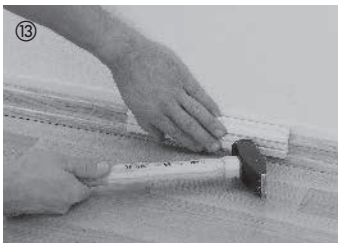
Be sure to remove all distance spacers once all boards are laid. Fasten skirtings (with or without clip system) to the walls – that's it.
