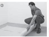
Always use 0.2 mm thick PE film as an underlay when laying your floor over floor screed This should overlap in the 30 cm impact area. Extend underlay up all walls. After having installed the skirtings cut underlay at the upper edge of the skirtings.
