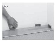
Align the boards of the first row with the groove side parallel to the wall, apply glue to the short sides (see fig. 5) and join the boards together. Fix them in place with spacers, leaving a gap of 10 to 15 mm between the floor and wall. Start the second row with the leftover piece of the first row. This considerably reduces waste (approx. 1% for longstrip).
