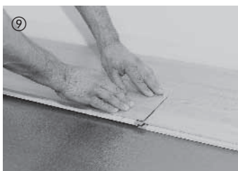
The board is then lowered in on the short side. Ensure here that the board is flush at the short side with the previously laid board. Pressure applied briefly to the side joint clicks in the board.
